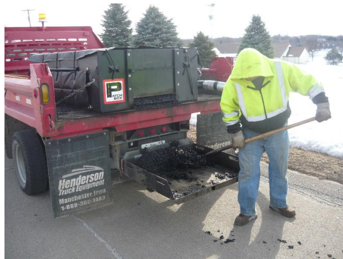
Figure 5 – Using the PatchCatch Tray for ergonomic shoveling
